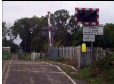
Help Point at level crossing
